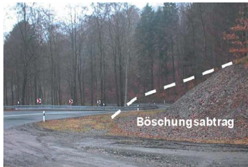
Figure 11: Removal of sight barriers in curves 11
