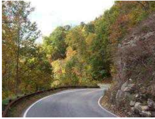
Figure 14: Dangerous obstacles in bends 13
