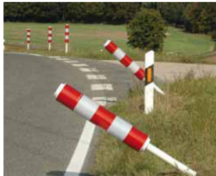
Figure 18: Guide posts made of flexible material 17
