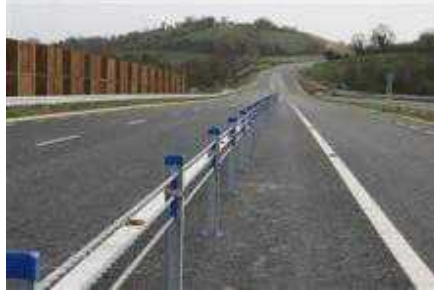
Figure 16: Wire rope barrier 15
